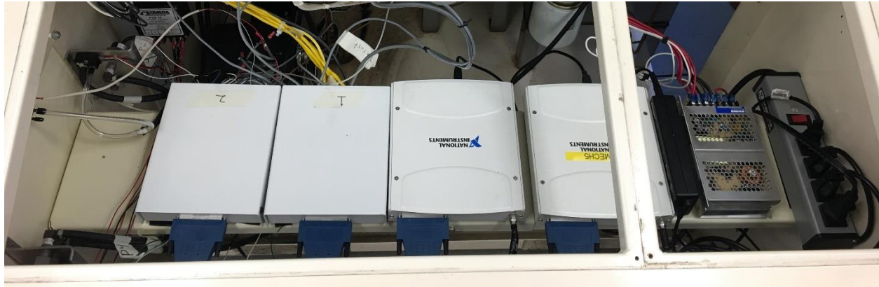
Figure 10. DAQ Components Installed
